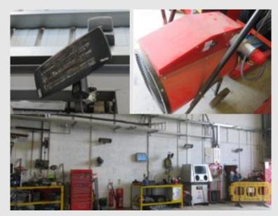
Consider install of insulated suspended ceiling, wall cladding and the use of radiant Ambirad type heating. The roof of the workshop regularly drips water from condensation in that building so insulation would be beneficial.
