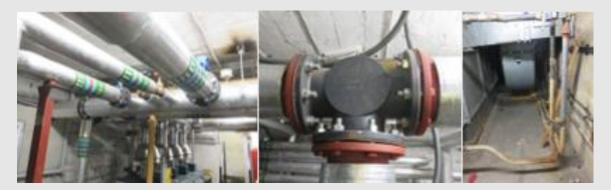
Similarly heating pipework serving the AHU should be lagged.
