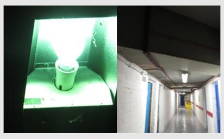
Red switches are left on 24/7. Install movement sensors on these fittings:
