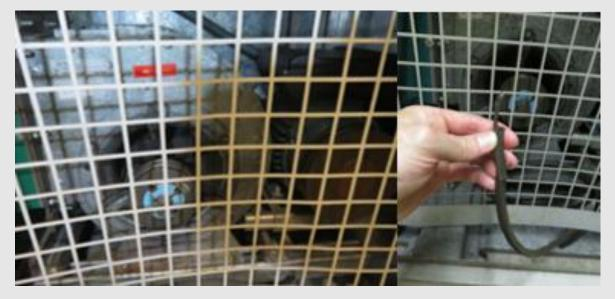
The belts themseves are a low quality/efficiency V belt and should be replaced with cogged belts for higher efficiency. The motor is old and if an investment could be made possible, it may be worthwhile replacing with a direct drive EC fan motor which, as well as being much more efficient, would not fail with the shearing of drive belts.
