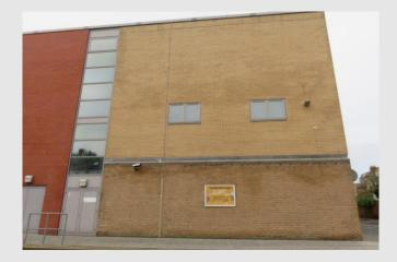
Given the heat loss potential at this site, this should be investigated. The age of the site makes it unlikely that insulation was installed at time of construction. There is no evidence of these walls being insulated as a retrofit. We would recommend and endoscope survey be conducted and if required, insulation pumped into the cavity.
