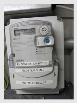
For the PV generation on this roof to have delivered 14,550kWh since installation on 5<sup>th</sup> February 2020 from a 19.5kWp array, is both impressive and further evidence (where it needed) of the fact that the 9.91kWp array at Plock Court is not delivering what it should be in a similar part of the country.
