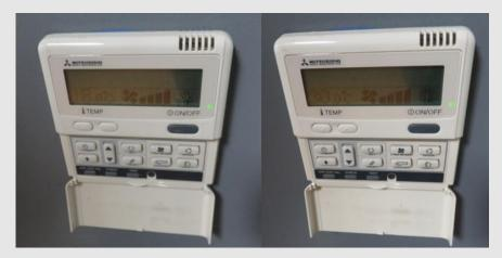
We would recommend locking these within a small range and by adjusting to 1C either side and adding this adjustment in 0.5C increments. Experience states that as long as staff are able to feel that they are in control, they do not need to move the dial particularly far. Heating for the site is managed on a Trend 963 BMS with the A/C units being managed by FM on a separate centralised Daikin controller.
